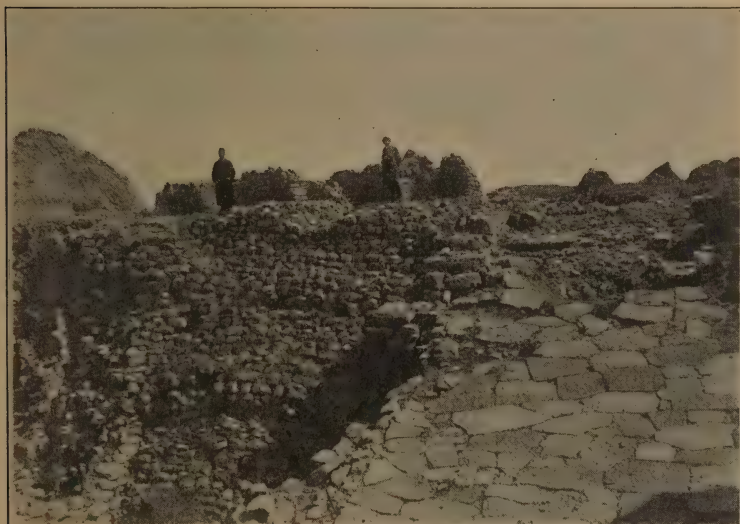
FIG. 337. — Paved road at Troy.
